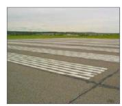
Threshold Markings indicate the beginning of the usable part of the Runway for aircraft landing. Threshold Markings are a series of solid white lines in groups that run parallel to the length of the Runway. The number of lines in a group and the total number of groups of lines is dependent on the width of the Runway.
