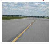
The Taxiway Center Line is a single solid yellow line on a Taxiway and is used to provide guidance for aircraft to taxi from the Runway center line to a point on the Apron where aircraft operational stand markings begin. The nose wheel of the aircraft is centered on this line to ensure that the main wheels are on the pavement and the wings will not make contact with any known obstructions.
