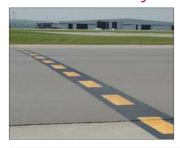
A Taxiway Intersection Marking consists of a single broken yellow line (e.g. at the intersections of Taxiways C and J). A Taxiway Intersection Marking is located at such a position that a holding aircraft or vehicle would not protrude into the intersecting taxiway strip. An aircraft or vehicle instructed to hold short of a Taxiway Intersection Marking must remain behind this line. These markings are co-located with Location/ Directional signs.
