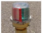
Runway Threshold Lights are two-sided lights, half red, half-green, and are used at the threshold of a Runway. The red half faces the Runway to indicate the end of the Runway and the green half faces the approach for the pilot to see when coming in to land an aircraft.
