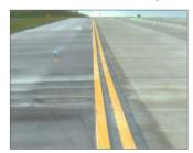
Taxiway Edge Lines consist of double solid yellow lines. The double solid yellow lines along with a series of single blue lights on a Taxiway are used to indicate the edge of the usable portion of the Taxiway. Paved surfaces outside the lines are not designed for aircraft.
