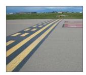
Runway Holding Position markings consist of two solid and two broken yellow lines across the width of a Taxiway with the broken lines closest to the Runway to indicate a Runway holding position.
