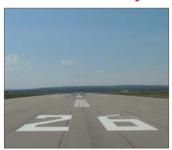
Each end of a Runway is numbered with the Runway Heading, in tens of degrees, corresponding to the direction of the Runway in relation to a magnetic compass. The compass of an aircraft will read 260 degrees when approaching the end of a Runway marked with the number 26. The numbers are painted in white and face towards the end of the Runway, YYC Runway headings are 08, 11, 17R, 17L, 26, 29, 35R, and 35L.
