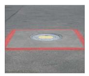
A red square indicates an underground fuel valve that is used when refueling aircraft. Parking is not allowed over or within 2 meters of Fuel Isolation Valve Chambers (Fuel Vaults).
