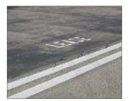
Lease Lines are two white (or yellow) parallel lines with the word "Lease" (or a company name). Lease Lines are used to outline the area of an Apron surface that has been leased to a company. An AVOP is not required for company employees or company authorized persons to operate vehicles, equipment or aircraft inside the leased area.
