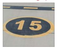
Geographical Position Fix Markings (also called 'Spots') are yellow circles with a number inside and a broken yellow line nearby. These 'Spots' are on the Apron near the exits to Taxiways and are used by Air Traffic Control (ATC) to help direct aircraft taxiing and aircraft under tow transition between the Apron and a Taxiway. The broken yellow line at a 'Spot' acts as a preliminary Hold Line for aircraft exiting the Apron.
