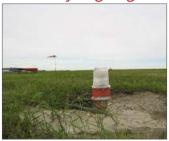
Runway Edge Lights are single white lights used along the edges of Runways. Runway 17L-35R has lights with a two-color head. The last 600 meters (2000 feet) of lights are yellow on one side and white on the other. The yellow lights act as a warning to pilots that the Runway is about to end.
