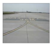
A Maximum Wingspan Marking is information denoting the maximum aircraft wingspan allowed in that area. The wingspan of an aircraft is always measured in a straight line, from wingtip to wingtip, independently of wing shape or sweep. The Maximum Wingspan Marking is located across the surface of a Taxiway/Apron Taxiway centerline.
