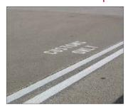
The CBSA Apron is marked with two parallel white lines with the words "Customs Only". The CBSA Apron outlines the airside parking area in front of the CBSA building on the North end of Apron VI. It is prohibited to drive through this area when an aircraft is parked in the CBSA area (Ref. 6.4). Vehicles can only enter the CBSA Apron when aircraft are present with specific authorization from CBSA.
