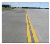
Apron Edge Lines are double solid yellow lines. Apron Edge Lines and the co-located single blue lights. Apron Edge Lines and the co-located single blue lights are used to indicate the edge of an Apron and the edge of a Taxiway. Paved surfaces outside of the Apron Edge Lines are not designed as weight bearing surfaces adequate for aircraft. Vehicles and equipment parked or operating outside of the Apron Edge Lines are NOT guaranteed safe clearance from aircraft.
