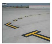
Aircraft Lead Out Lines are a single broken yellow line and are used to guide the aircraft as it taxis out of its Ground Loading parking position. This is the route an aircraft takes when leaving a Ground Loading Operational Stand under power.
