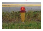
Single red lights are sometimes used to indicate the end of a paved surface.
