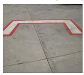
A Bridge Staging Box is a white or red U-shaped marking and is used to indicate where the bridge wheels may be pre-positioned, while still providing clearance for specific aircraft entering the operational stand. The outer red line indicates No Parking in this area.
