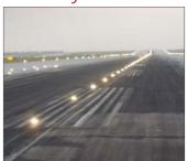
Runway Center Line Lights are inset white lights that run along the Runway center line with directional red lights at the extremities of the Runway. The last 300 meters of the center line lights are red, and the lights between 300 meters and 900 meters alternate between red and white. This system of red and white lights act as a warning to pilots that the Runway is about to end. Runway Center Line lights are located only on Runway 17L-35R.
