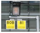
The A-VDGS (Ref. 1.3 for definition) provides aircraft with accurate guidance into the gate and real time data through the display unit. The system allows aircraft to dock safely thereby allowing passengers to deplane without the need for marshallers, thereby minimizing the risk to ground personnel during lightning events. The A-VDGS is intended primarily for use during lightning events, and may be used at anytime, at the discretion of the air carrier/operator.
