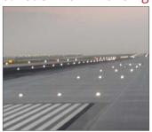
Touchdown Zone Lights are a series of three inset parallel white lights that run between the Runway center line and the Runway edge for 900 meters. Touchdown Zone lights are available for use in low visibility conditions to mark the aircraft landing/ touchdown zone. Touchdown zone lights are located only on Runway 17L-35R.
