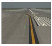
Rapid Exit Center Line lights are a series of inset alternating green and yellow lights. Rapid Exit Center Line lights mark the high-speed exits from a Runway to a Taxiway. The inset lights are two-directional so that the alternating colours show only when exiting the Runway and only if the lights are green from the Taxiway onto the Runway. Rapid Exit Center Line lights are located only on Runway 17L-35R.
